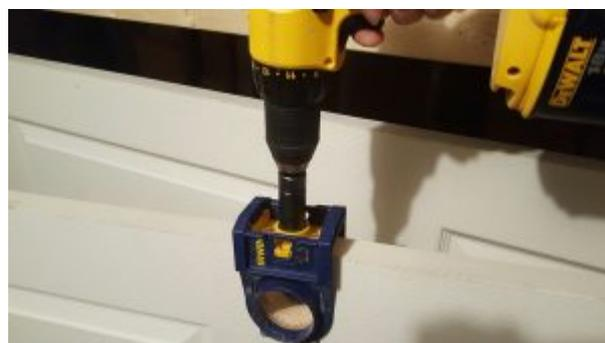
6. Now that you have your holes in place remove the guide and put the router latch guide on the side. Next, switch out the hole saw for the router bit and router out the template. Remove the template and use the chisel to remove the excess material, now making it flush.
