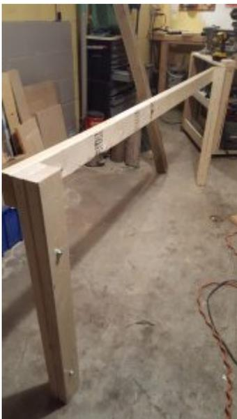
9. Now is the time to attach the front and back legs together. Your top should be 17.5" wide in total, and you do not want too much of an overhang in the front and the back.
