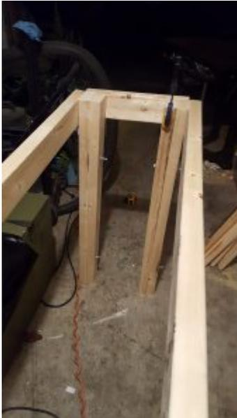
10. You also need to put in a blocking piece just above the bottom Hex Bolts on the legs to give the legs support down there. This is where the left over cut pieces are going to come into play. With 17" total you need, minus the front & back trim and the legs thus leaving you with an 8" piece on either side. Screw and attach this board in, however you may need to counter sink it since you are going through 2 pieces of 2"x4"s (legs)
