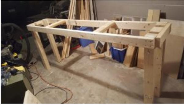
11. You also need to put in a blocking piece just above the bottom Hex Bolts on the legs to give the legs support down there. Now, this is where the left over cut pieces are going to come into play. With 17" total you need to minus the front & back trim and the legs. This should leave you with an 8" piece on either side. Screw and attach this board in, however you may need to counter sink it since you are going through 2 pieces of 2"x4"s (legs)
