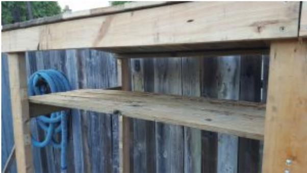
6. Use 2x4's as Diagonal supports between the studs. As a result you will notice a huge difference in strength of the shed after doing this.
