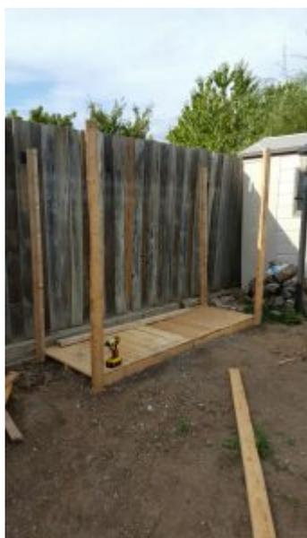
4. Make the start to your roof Using 2x4's in between the studs, as well as the the frame on one side for the Kindling Shelf.
